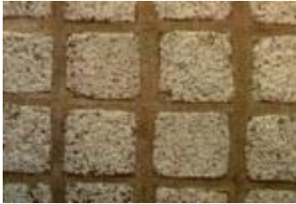
'Fine Picked' - also known as 'Bush Hammered'. Fairly smooth, good non-slip surface.
